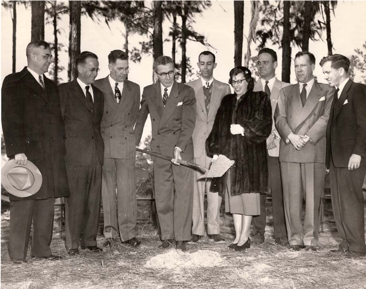
Jan. 25, 1953 – Groundbreaking for expansion of the original building
