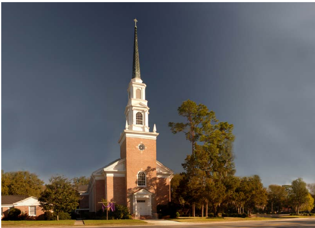
Lakewood Presbyterian Church, 2009
